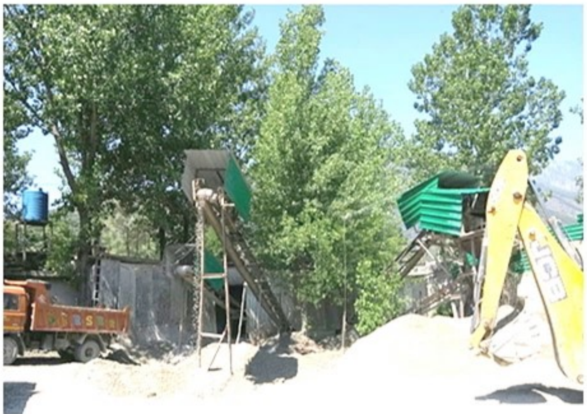
Photograph 02 (c & d): Stone Crushing section under Sheet Cover/Shed behind the conveyer.
