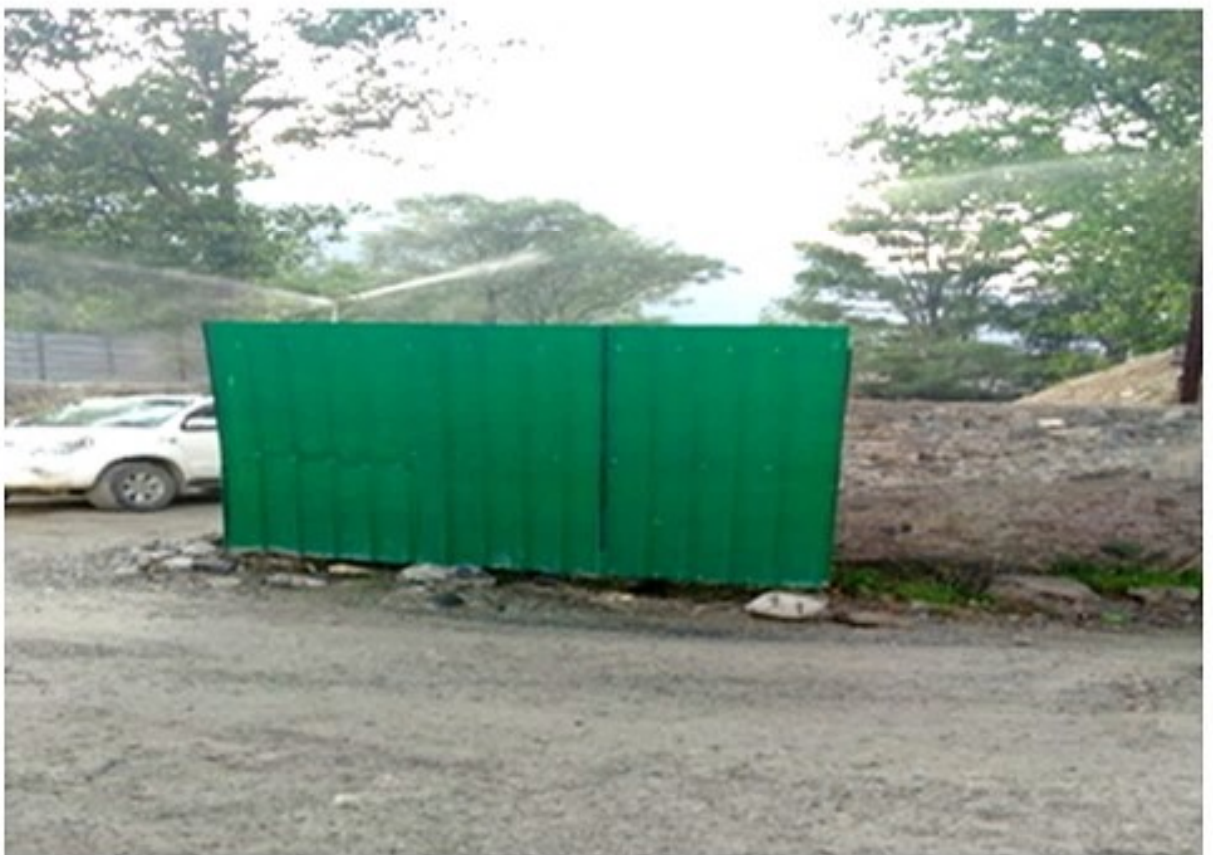
Photograph01 (a.&b): Entry of crusher: wetting of road and Wind breaking wall.
